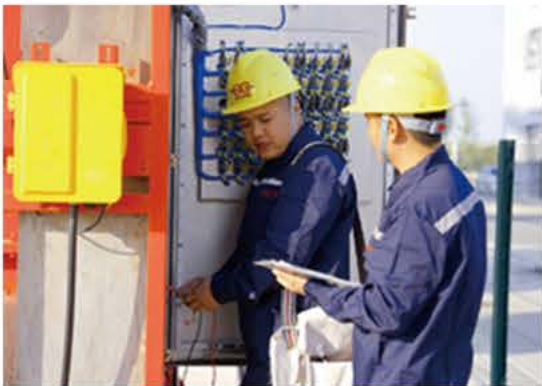
Dedicated and Regular Inspections
